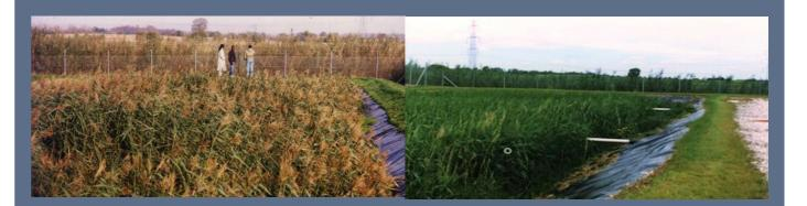
In the sludge mineralisation beds or root-zone, the dry matter is dewatered and mineralised so that the sludge amount is re-duced to 2-4% of the original amount.
